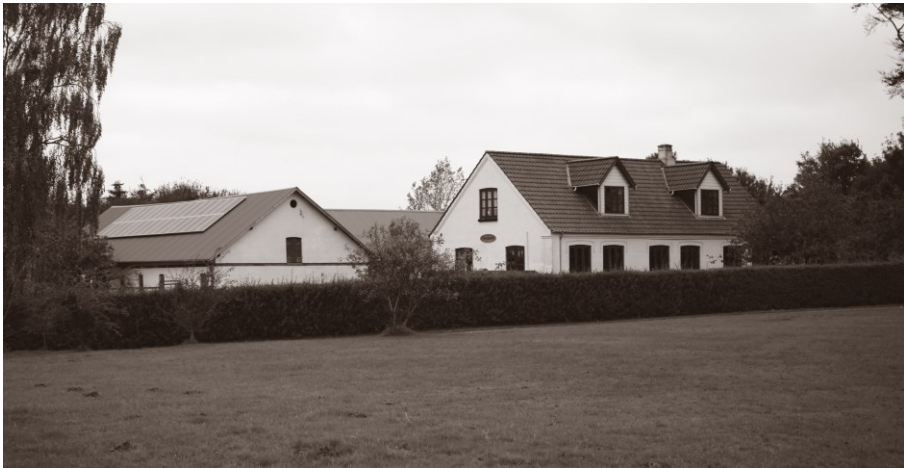
Parisgård i Over Barrit, 2015.
